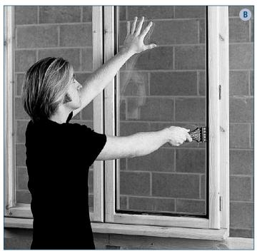
5. Check that the unit fits into the frame and can be centralised when standing the unit on setting blocks so that there is a minimum 5mm edge clearance at the bottom of the unit. The spacer bar should ideally be level with the sightline or slightly below it (see picture B).
