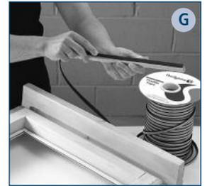
7. Align the bead blocks (if required) with the front edge of the bottom rebate platform no more than 50mm from either end and not more than 150mm apart (where the pencil marks should already be). A minimum of 2 blocks must be used for the bottom bead.
