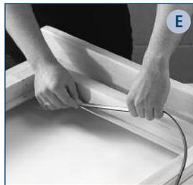
3. Start the application of the second length of Foamsekre® XD to the side rebate by forming a butt joint against the length already positioned, taking care to line the edge of the second length of tape with the sightline (see picture F). Apply the tape to both sides and then the top. Remove the backing paper.
